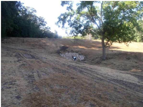
2010 Flood Repair (Pond Repair)
