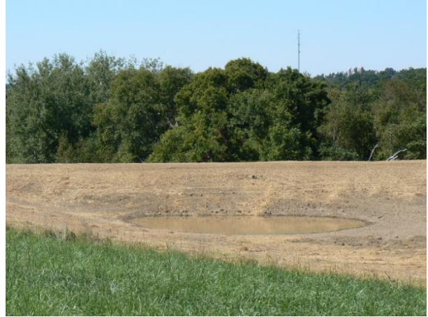
Grade Stabilization Structure (pond)
